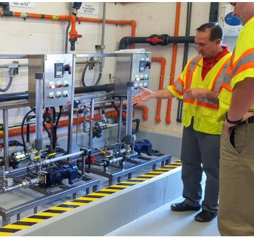
into DC drives with programmable logic. If the pump broke down, the drive would have to come out as well because it could no longer communicate with their control board properly. The City had a "trailer full" of metering pumps actively being worked on at any given time, to ultimately be disposed of. Since the City was already using PC pumps that required very little work for sludge, Rick suggested to Director of Operations, Poonam Kalkat, who
